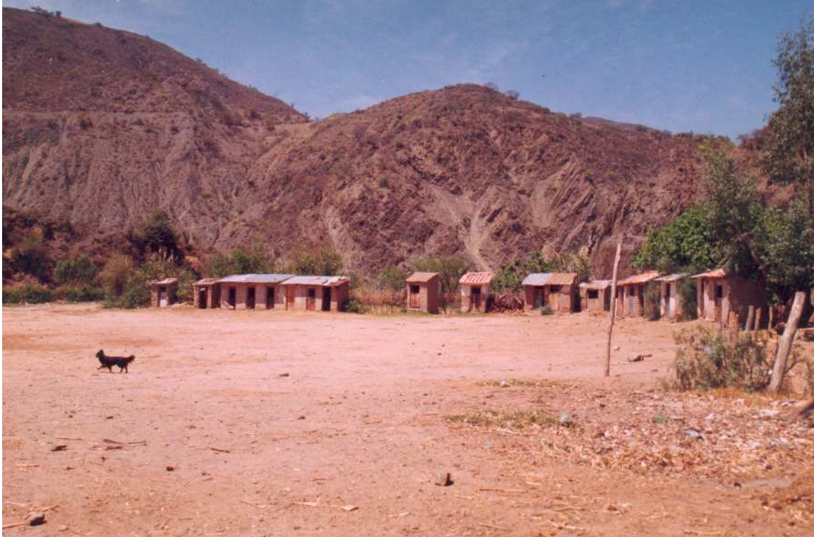
Figure 6.3 Latrines in Yotala, constructed with LPP-funds.
