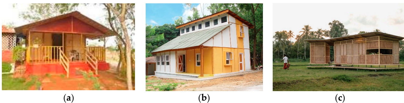
Figure 5. (a–c) Example homes in India. (a) House in Aleru. Source: Bamboo House India [25]; (b) Earthquake resistant house with bamboo frames and panels [26], (c) Modern bamboo house on stilts, in Kerala. Source: NO Architects [27].
