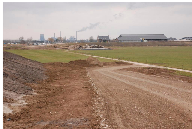
Fig. 2. Old and new: terp construction in the Overdiepse polder.
