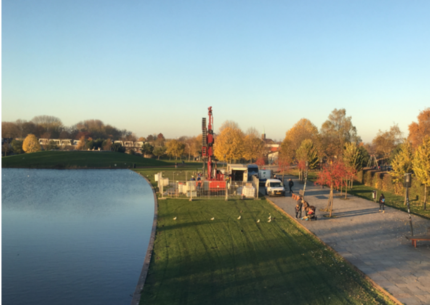
Figure 2.4: Sonic drill in operation in the Griftpark.
