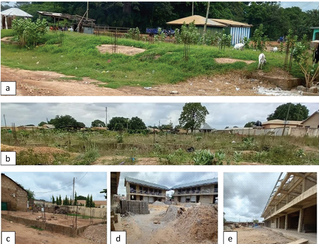
Figure 5. Field photos of incremental housing development in Wa (a–c) and ongoing construction at the central business district (d and e). Source: Authors, July 2021.
