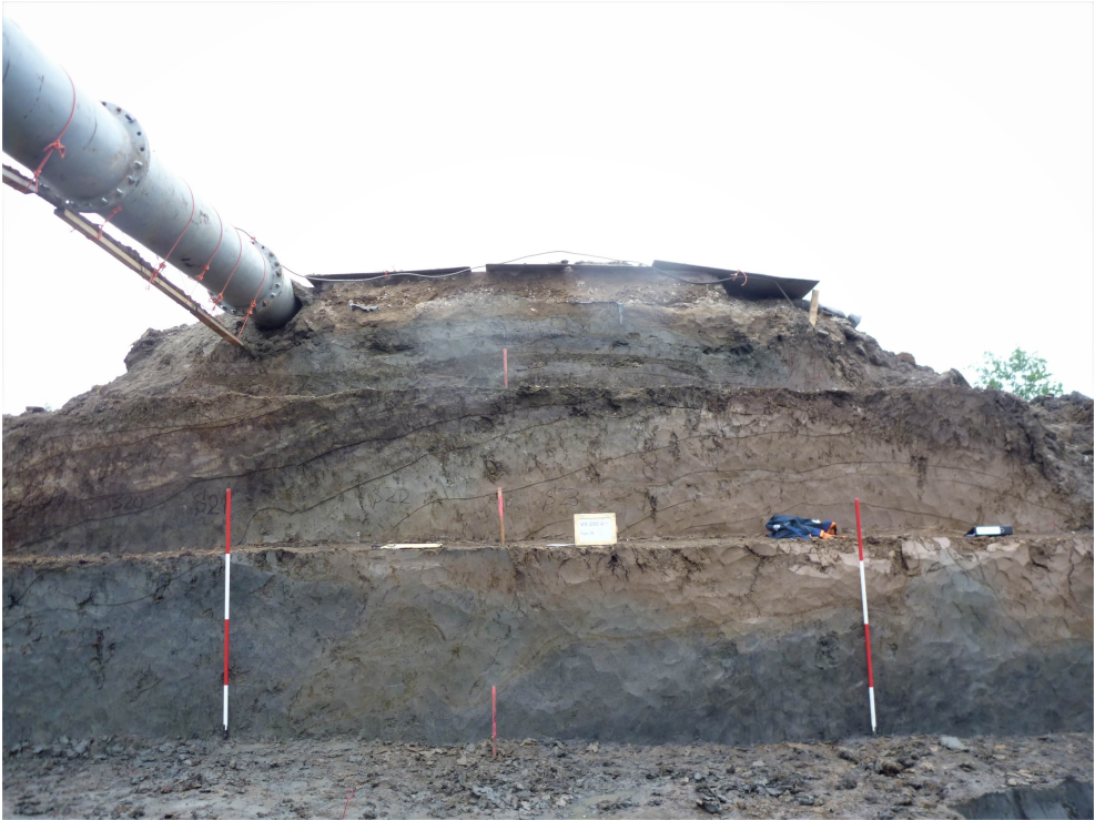
Figure 4.1 Example of historical dike buildup as seen in the archaeological excavation in Vlaardingen (schematized in Figure 4.5, see Appendix A.1 for source). The variation in color is a first indication of variable material textures, which are mostly variations of clay-silt mixtures in this dike, with sandy to gravel deposits on the top, which form the road foundation.
