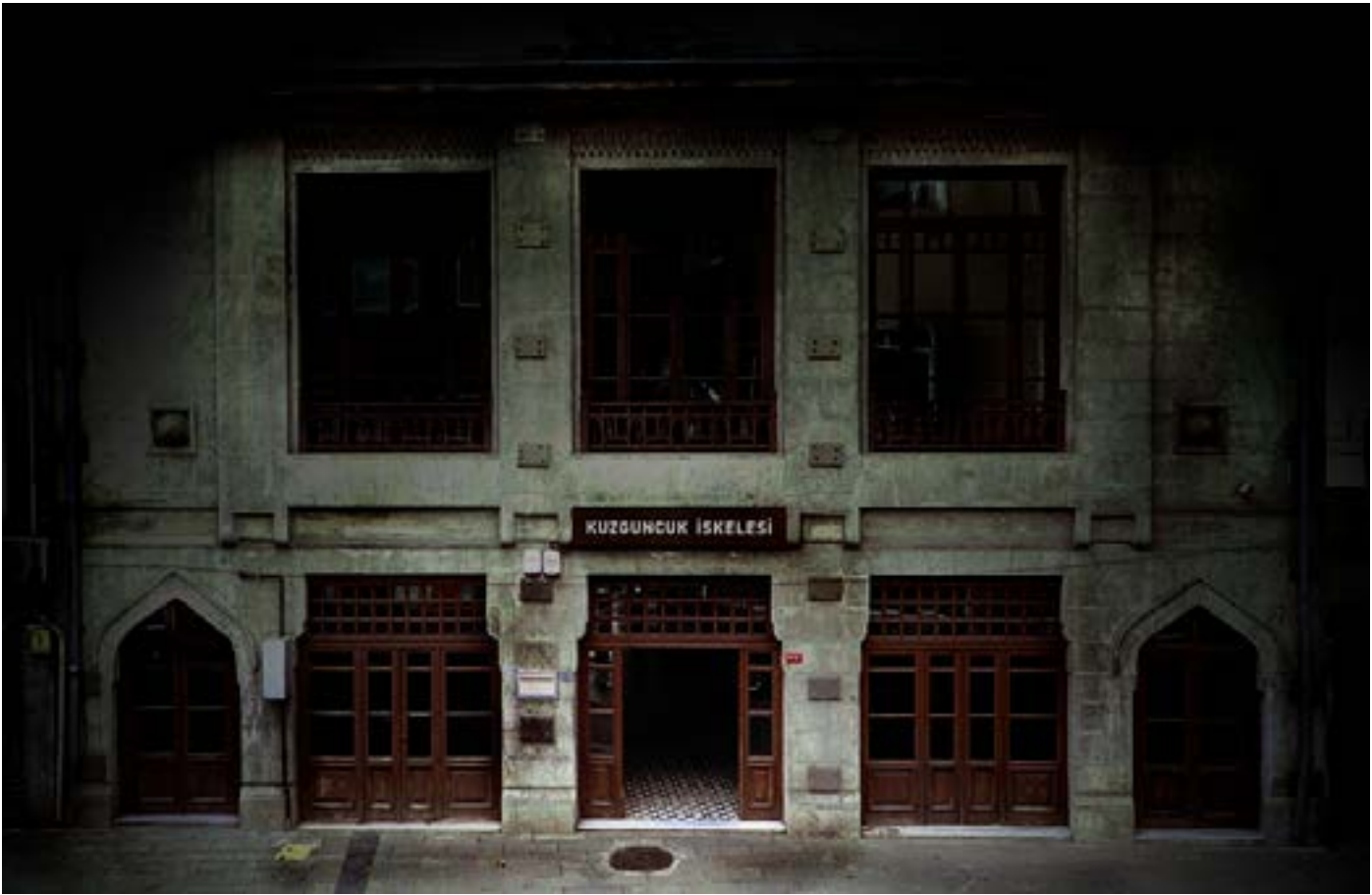
■ Figure 1. Kuzguncuk Pier's facade, Istanbul. Photo courtesy Yoğunluk Art Collective
