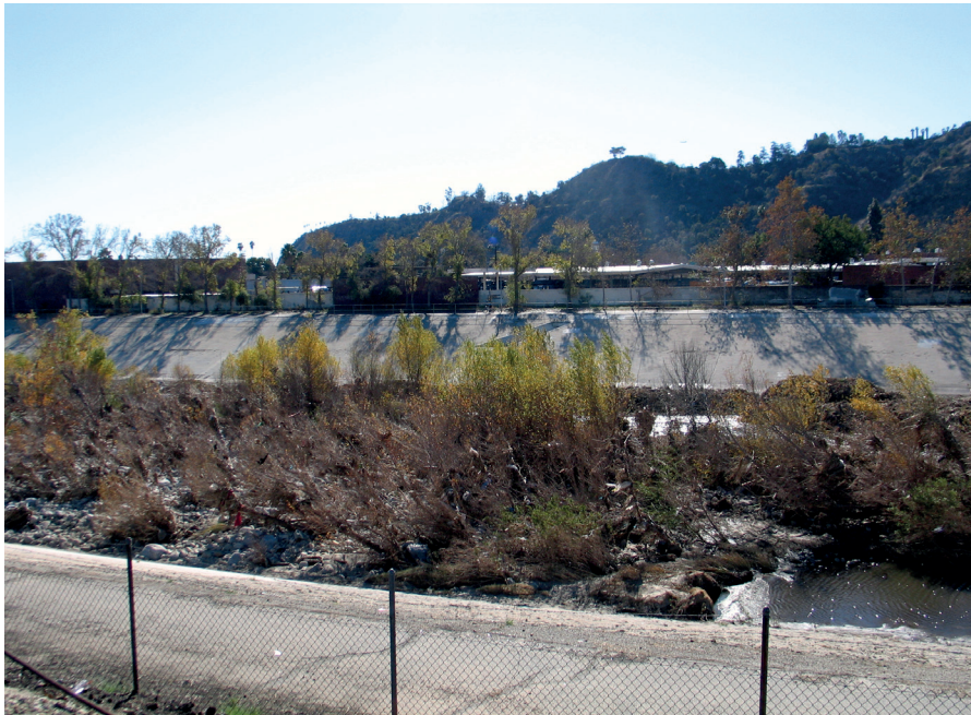
FIGURE 4 The Los Angeles River in the Glendale Narrows (photo by Valentin Meilinger, 2018)
