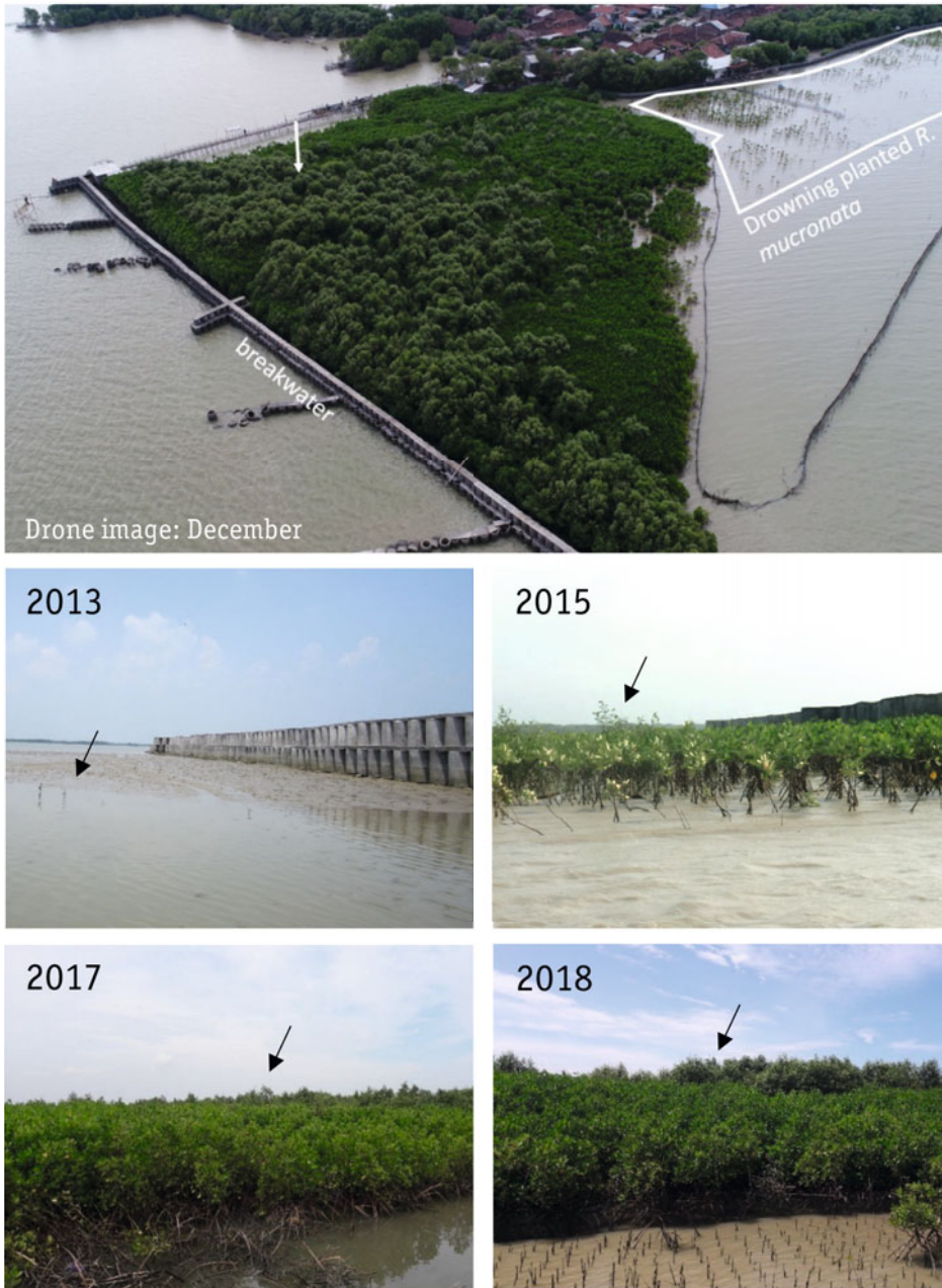
Figure 4-9: Top: Bird's-eye view of the breakwater seaward of Wonerejo, Demak in 2017 (drone image courtesy of CoREM-UNDIP). The white arrow indicates the direction of the picture time series. The time series show the development of a mudflat after construction of the breakwater in 2012, followed by natural colonization in 2013 and subsequent planting of R. mucronata in 2014. Note the relative height difference in all pictures of the naturally colonized A. alba trees (black arrows) versus the surrounding planted R. mucronata trees (2015-2018).
