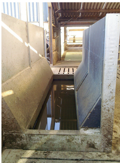
Figure 2.4. Wisconsin footbath design. Note the 28 cm high kerb which encourages more frequent, shortened steps for added plunges, as well as reducing solution loss (i.e., kickout). The solid sides promote better cow flow while again reducing solution loss. The 60 cm wide footwell is just wide enough to allow cows to walk comfortably, but allows for the length of bath to be extended to 3.7 to 4 m without inflating the volume excessively. The footbath is set at the existing floor level so the cow can step in and out with confidence.
