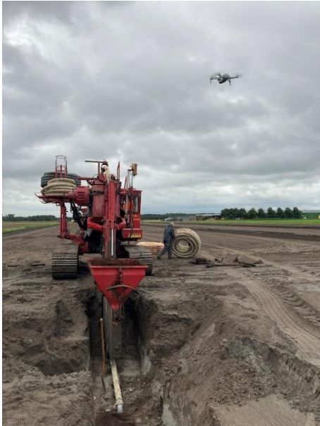
Figure 1-7 Construction of drains covered with ICS
