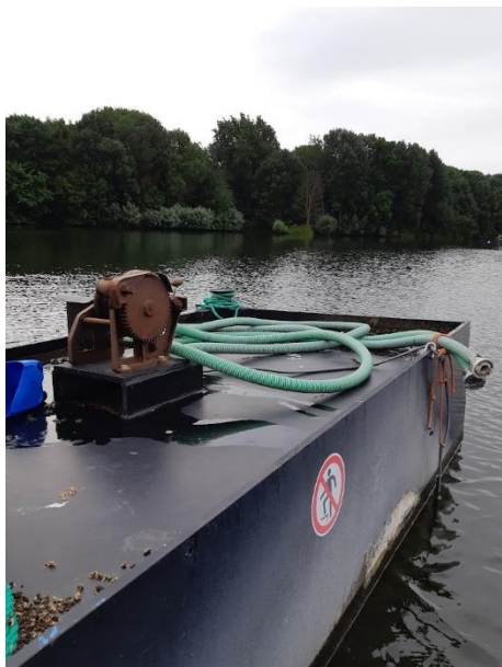
Figure 6-2 ICS filter in a lake. The filters are two big-bags with 1m 3 of ICS each and a pump in the center, the filters are 2 m below the surface. The water enters from all sides of the big-bag and the hose is the outflow of the filter.
