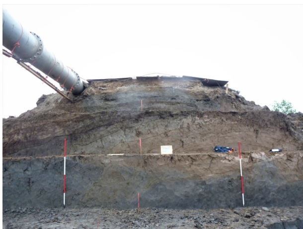
FIGURE 1 Example of historical dike buildup as seen in the archeological excavation in Vlaardingen (schematized in Figure 4, see Appendix A for source). The variation in color is a first indication for variable material textures, which are mostly variations of clay-silt mixtures in this dike, with sandy to gravel deposits on the top, which form the road foundation
