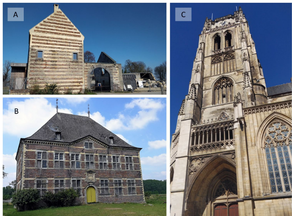
Fig. 6 A Ferme de Caestert (Ternaaien, BE), located south of Maastricht, with horizontal layers of Maastricht Stone (white) alternating with horizontal layers of brick masonry (red) typical of local renaissance architecture; B Infirmierie , Herkenrode Abbey Hasselt, Maastricht Stone in combination with blue stone (Carboniferous limestone) and brick, typical of local renaissance architecture. C Gothic Our-Lady Basilica with belfry tower in Tongeren (BE) as part of a World Heritage ensemble (Belfries of Belgium and France), built in Maastricht Stone
