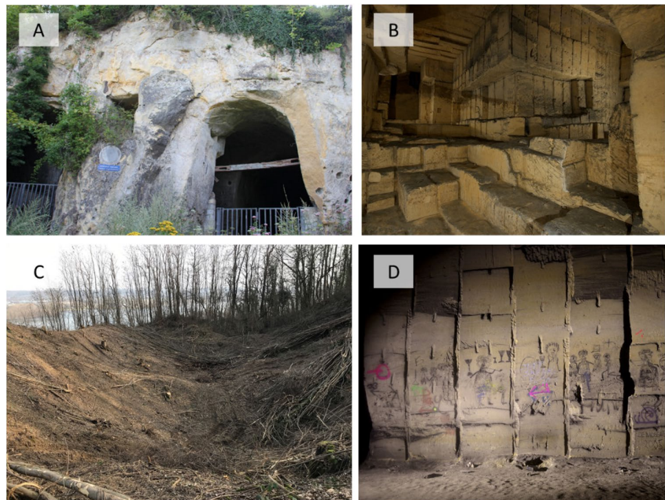
Fig. 5 A Entrance of the underground quarry Grootberg (Kanne, BE) visible in the surficial landscape of the valley-flanks. B Subterranean landscape of the quarry Grootberg where the excavation in blocks is comprehensible. This gallery has not been transformed for secondary purposes ©VZW Hulpdienst Groeven. C Surficial landscape above an old collapse of an underground gallery of the quarry Caestert (Caestert, NL), clearly visible after tree felling. D Underground gallery of quarry Ternaaien Beneden (Ternaaien, BE), with historical graffiti on the block-shaped wall (black drawings) vandalised by modern graffiti (colored tags) ©VZW Hulpdienst Groeven
