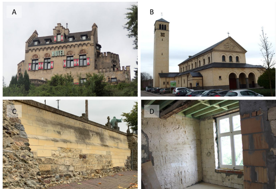
Fig. 7 A Former Villa Zuyderhorst in Berg en Terblijt (NL), constructed in Maastricht Stone in 1918 in English Gothic Revival style. B Saint Lutgardis, patroness saint of Flanders region sanctuary in Tongeren, designed by architect Jos Ritzen and constructed in 1954, clad inside and outside in Maastricht Stone from the two last active underground quarries in Kanne and Zichen (Dusar et al., 2017). C Church wall around Brigida church in Noorbeek (NL) with replacements in new blocks of Maastricht Stone. D Maastricht Stone as inner wall in a private dwelling in Riemst (BE), visible after removing plaster during renovation works
