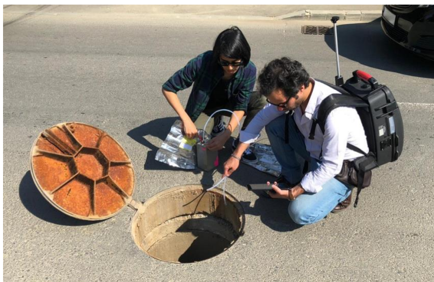
Figure 3.S3. Sampling a known pipeline leak for source signatures. Residential utility manhole on Drumul Potcoavei (Horseshoe Road) (44.505°N, 26.133°E), 410 meters from the Bucharest city border. Manhole was opened with the assistance of the local gas company, and confirmed a pipeline leak. Fernandez, J.M. collects air samples for the analysis of CH 4 mixing ratios, \delta D-CH_4 , and \delta^{13}C-CH_4 (via bag pump and FlexFoil sample bags). Maazallahi, H. measures real-time CH 4 and C 2 H 6 mixing ratios for C 2 :C 1 ratios using a Picarro backpack Gas Scouter TM G4302.
