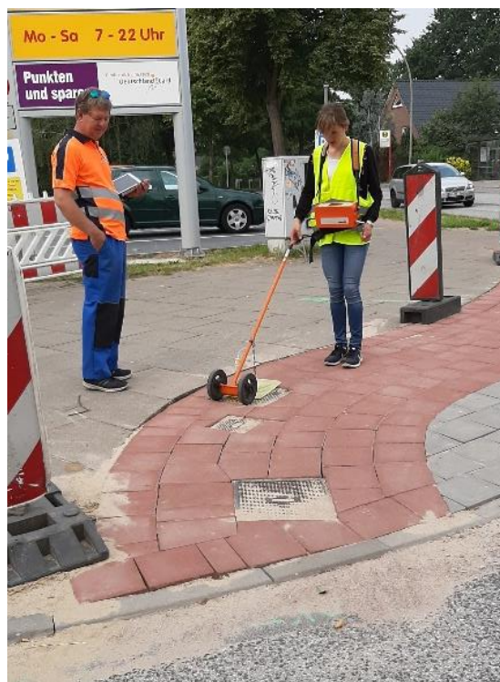
Figure 2.S18. Leak detection operation by GasNetz Hamburg
