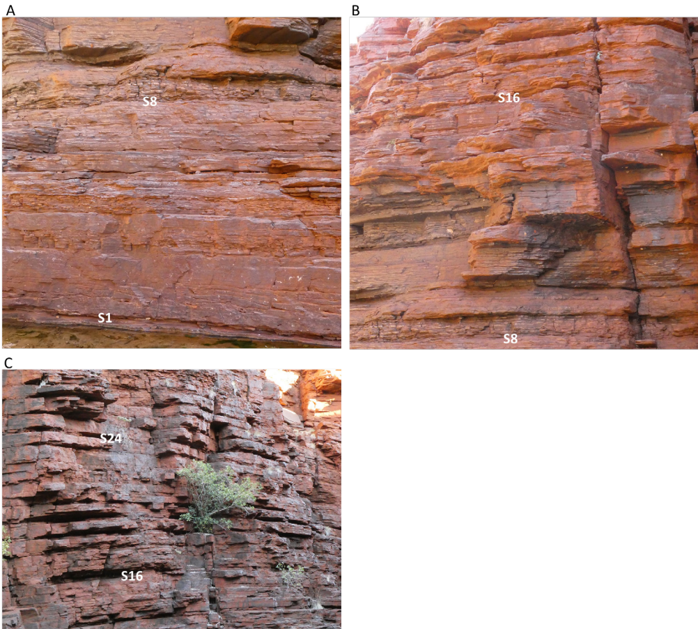
Figure S3. Photographs of the logged shale-BIF alternations at Joffre Falls. (A - B) Bottom section (S1 – S14). The alternations at the base of the gorge have a more blocky appearance, which we suspect is mainly related to a difference in weathering compared to higher up in the sequence. The rocks at the base of the gorge are more frequently polished by river water resulting in a fresher surface exposure. (C-E) Middle section (S14 – S49). Note the distinct shales S16, S18-S19 and S23 – S29 surrounded by intervals with weaker shales. (F - G) Top section (S49 – S57). This section is relatively far away from the waterfall and so the rocks have been more affected by chemical weathering, producing larger and more gradual relief changes from ‘BIF’ to ‘shale’. This is incorporated in the logs as transitional ‘platy’ intervals between the shale and BIF units occurring in BIF 51 to 56 (Fig. S4).
