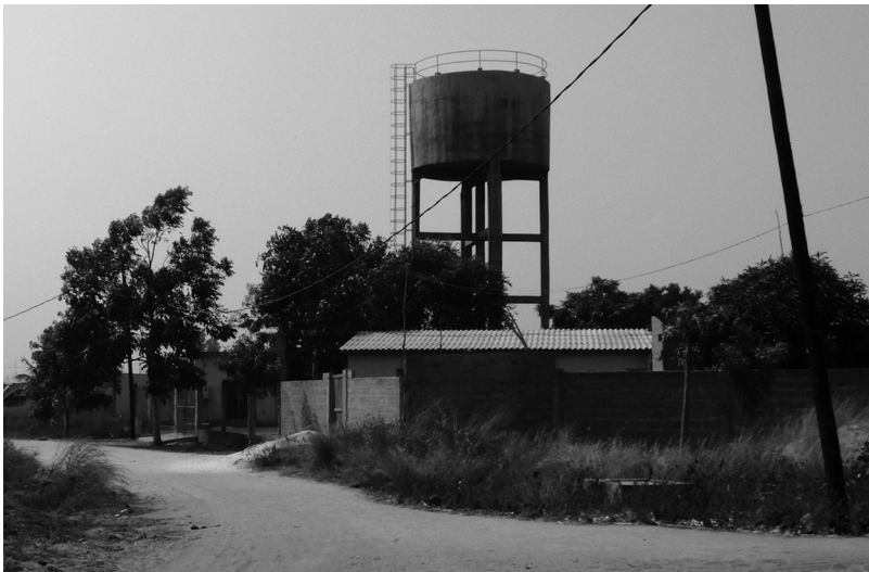
FIGURE 3.4 The water tower, a symbol of the resettlement site. source: authors, 2017
