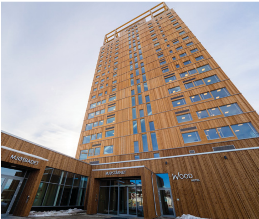
Figure 4 The 85-meter-high Mjøstårnet in Norway. The building’s structure is composed of both glued laminated timber and cross-laminated timber Source: The photo is provided by Moelven 2019
