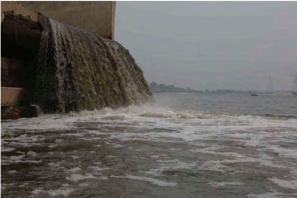
Figure 1. Sewage treatment plant outfall at Jajmau.
