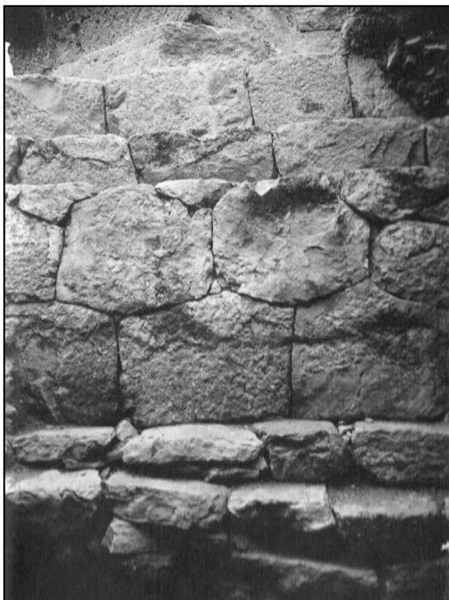
Figure 65 – Lesbian masonry of the Early Archaic Retaining wall.
