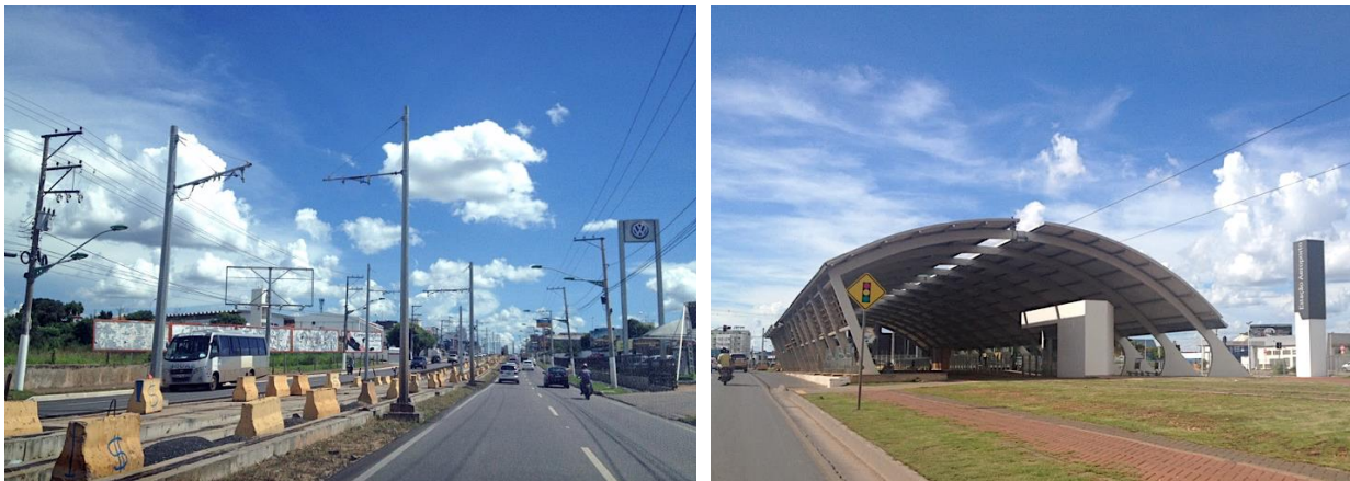
Figure 14: The unfinished VLT in Cuiabá (left) and one of many unfinished stations (right)
