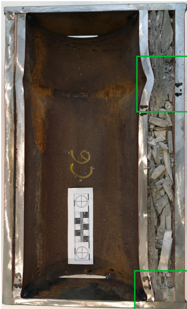
Fig. 18. Axial cross section through the dent at 1.0 m (top-most dent) and one half of the dent at 1.3 m (bottom-most dent). We observe generally fragmented and poor cement away from the dents. At 1.1 m and 1.3 m, the cement appears to have improved cohesion compared to the initial condition seen away from these positions.
