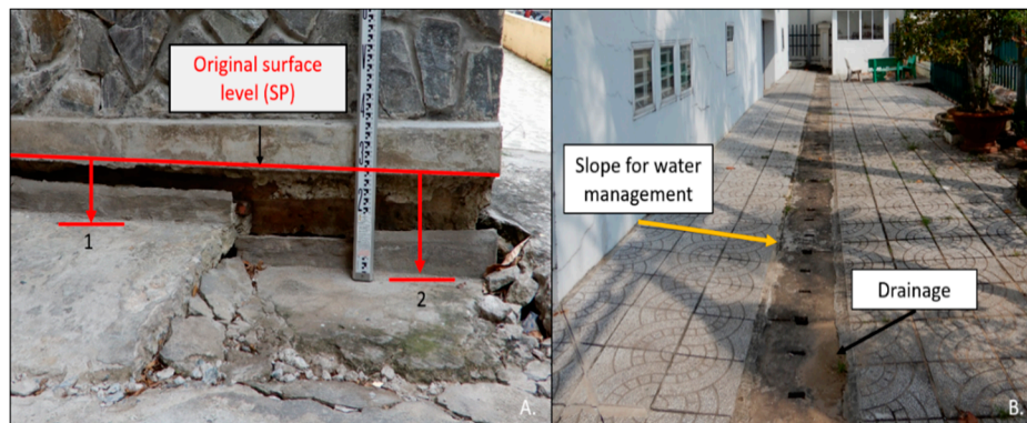
Figure 7. (A) Example of local variation in current surface level causing uncertainty in determining the actual offset caused by subsidence (1 or 2). (B) Sloping surface constructed as a water management measure instead of resulting from subsidence.
