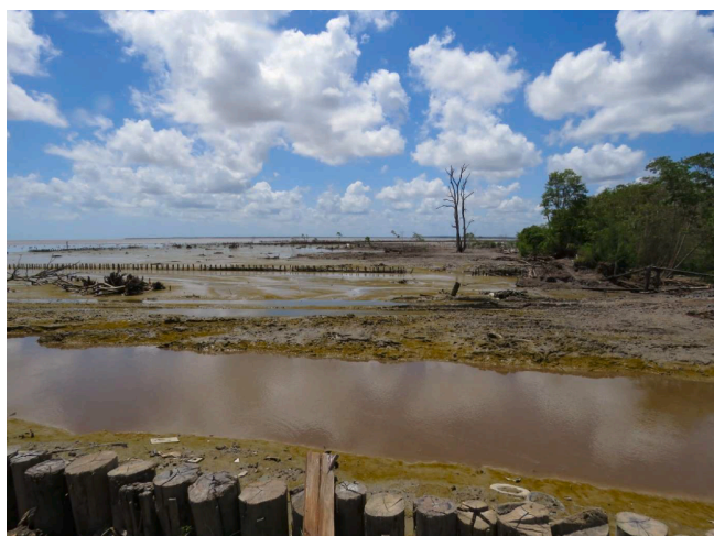
Fig. 3b. Example of renewed accretion after coastal erosion at Weg naar Zee in Suriname (Photo: Steven M. de Jong, June 2019).
