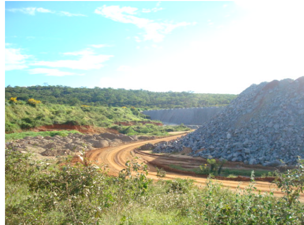
Figure 1b. View of the constructed solid waste deposit in 2008 (sterile soil on the left, leachate ore in the center, and sterile rock on the right).
