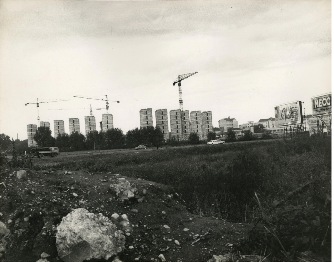
Figure 2: Carlo Cisventi, Milan: Residential Neighbourhood under Construction, c.1960. b/w photographic print, silver bromide gelatine. 230 × 291 mm paper. CSAC Università di Parma – Archivio Cisventi. © CSAC Università di Parma.
