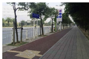
Shared bike paths Shared bike paths are on-sidewalk bike paths that have been developed specifically to differentiate the path from the common pedestrian sidewalks with colored pavement or markings.
