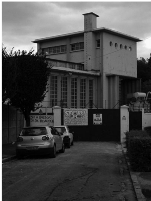
Figure 2: Power substation in Clichy-sous-Bois (photo by the author).
