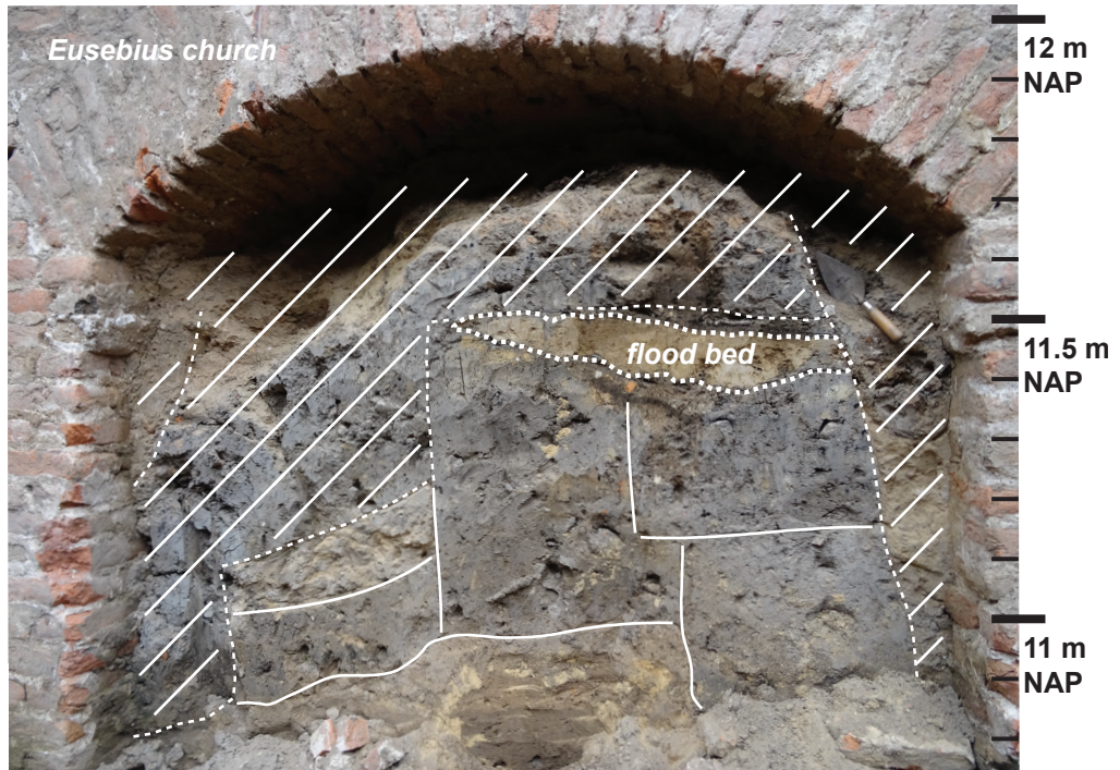
Fig. 2.7. Complex anthropogenic stratigraphy in a pocket of ground between foundation structures of the Eusebius church southern nave face. No layers in this profile react with hydrochloric acid, except for the light-coloured yellowish deposit indicated as a flood bed. The hatched layers fill the pits dug to construct the brick columns and arch during the church expansion and rebuilding phase between circa 1450 and 1550 (den Hartog and Glaudemans, 2013), supporting a late fourteenth-century age for the flood bed. The present street level at this location is approximately 13 m NAP.
