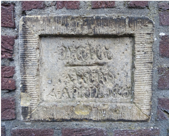
Fig. 3.20. A flood mark in Wijk bij Duurstede. The inscription reads 'WATER- STAND A: APRIL 1845'. The horizontal line in between the words 'WATER' and 'STAND' represents the maximum water level.
