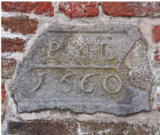
Fig. 3.9. Stone in the city wall of Leerdam that resembles a flood mark, as it depicts both a year and a horizontal level. However, it likely does not indicate an actual water level, as no flood occurred in 1660. Instead, the stone refers to an agreed-upon water level for piercing a dike during flooding in order to protect one polder area at the cost of another (this agreement was still in use circa 150 years later; Ewijk, 1809). Note that major floods occurred in 1651 and 1658, and the mark may relate to a water level reached in those years, although it is positioned remarkably high (above the water level reached during the major flood of 1809).
