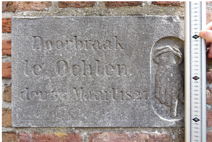
Fig. 3.2. Example of a flood mark in Culemborg. The stone informs on the water level (base of stone as indicated by the index finger of the depicted hand), and on the location and date of dike breaching (Ochten, 3 March 1827).
