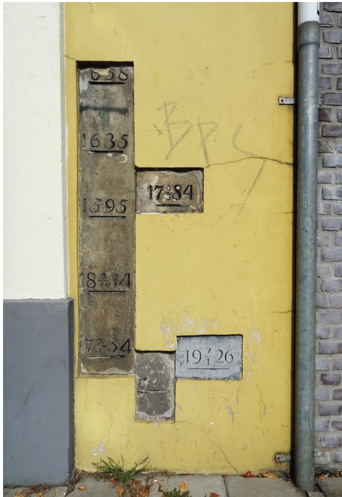
Fig. 3.6. Example of a series of flood marks in Deventer. Note that the mark of 1595, the oldest recorded year, is precisely in the middle of the main stone. Thus, the stone was very likely placed in that year, with the intention to record future extreme flood levels in the space above and below. Further note that for some years, the month and day of flooding are indicated in between the century and decade numbers. This way of denoting the date of flooding has been observed for a number of marks across the delta.
