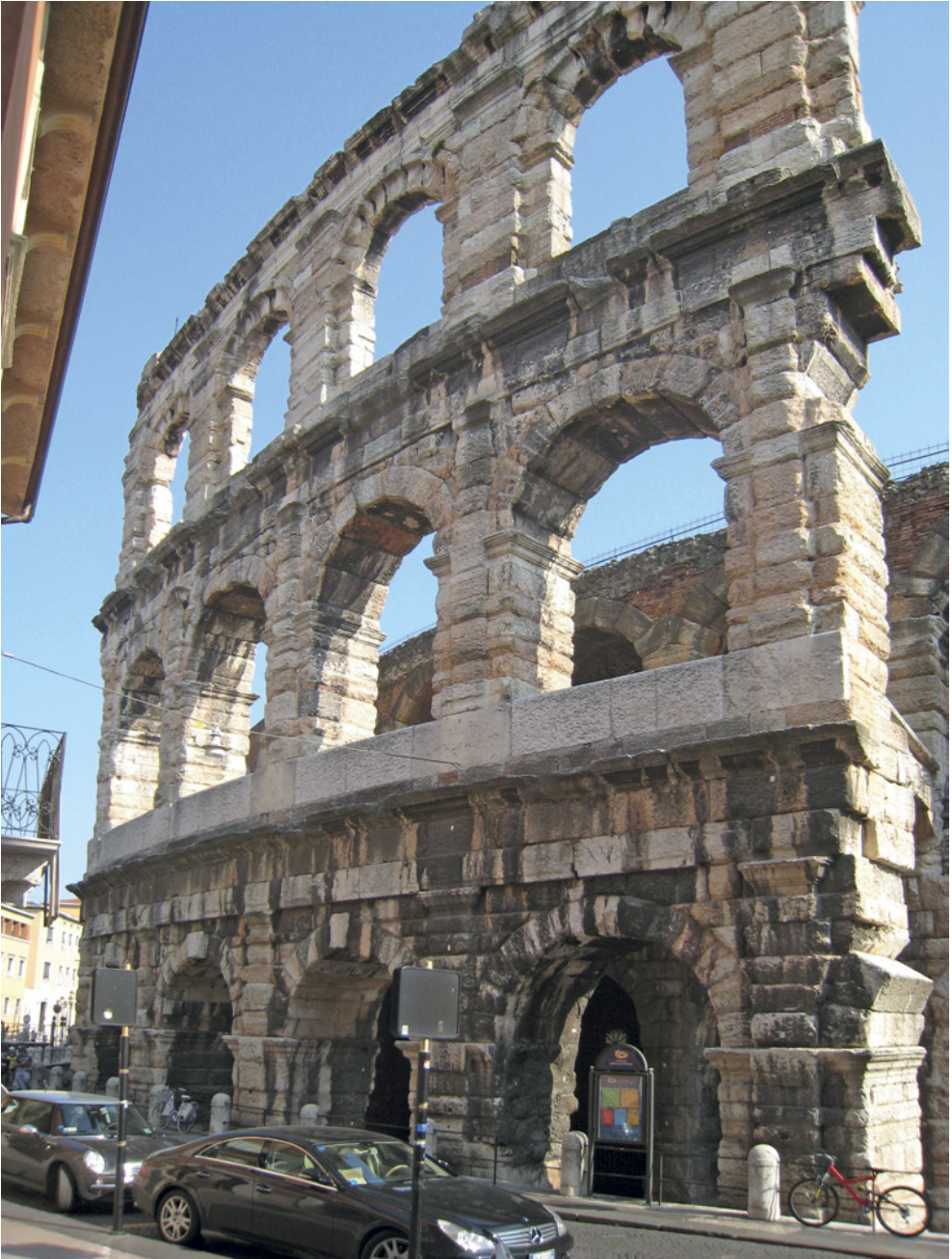
FIGURE 3.3 Arena of Verona (first half of the first century AD), remains of the outer wall IMAGE © AUTHOR
