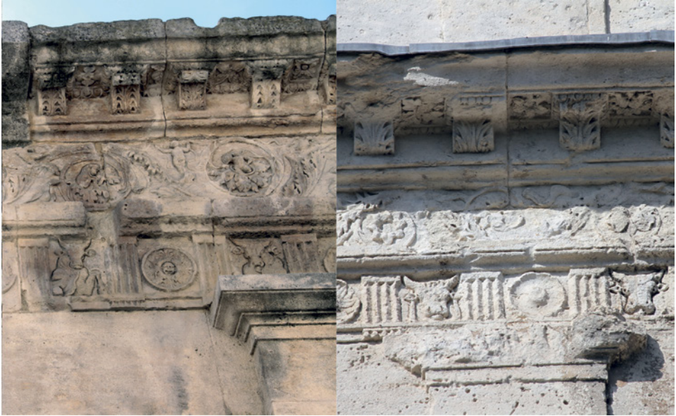
FIGURE 8.5 Left: Doric entablature of the “Arcade of Mercy” at the theatre of Arles. Right: Doric entablature (second level) of the “Tower of Roland” of the same theatre
