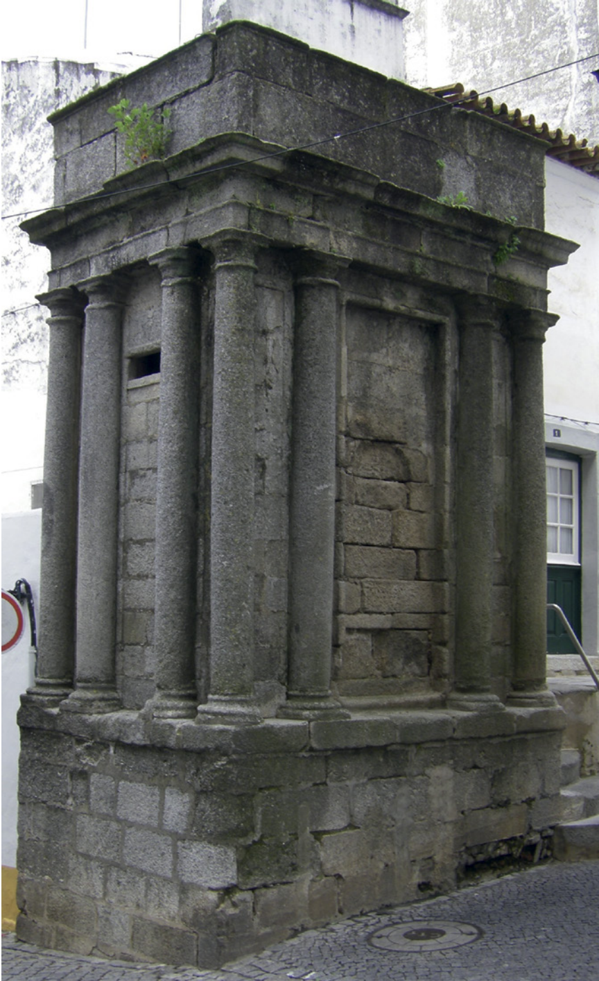
FIGURE 5.9 Water reservoir, part of the aqueduct of Água da Prata, Évora IMAGE © NUNO SENOS
