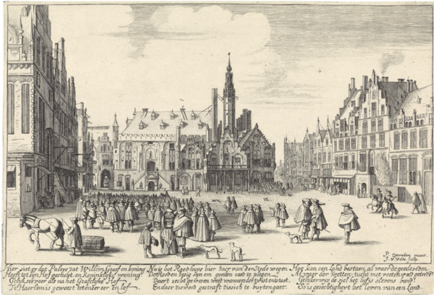
FIGURE 16.2 Market square and town hall of Haarlem before its transformation of 1630–1633. Etching by Jan van de Velde II after Pieter Saenredam. From: Samuel Ampzing, Beschryvinge ende lof der stad Haerlem in Holland (Haarlem: 1628). Etching and engraving, 16.1 × 23.8 cm IMAGE © RIJKSMUSEUM, AMSTERDAM
