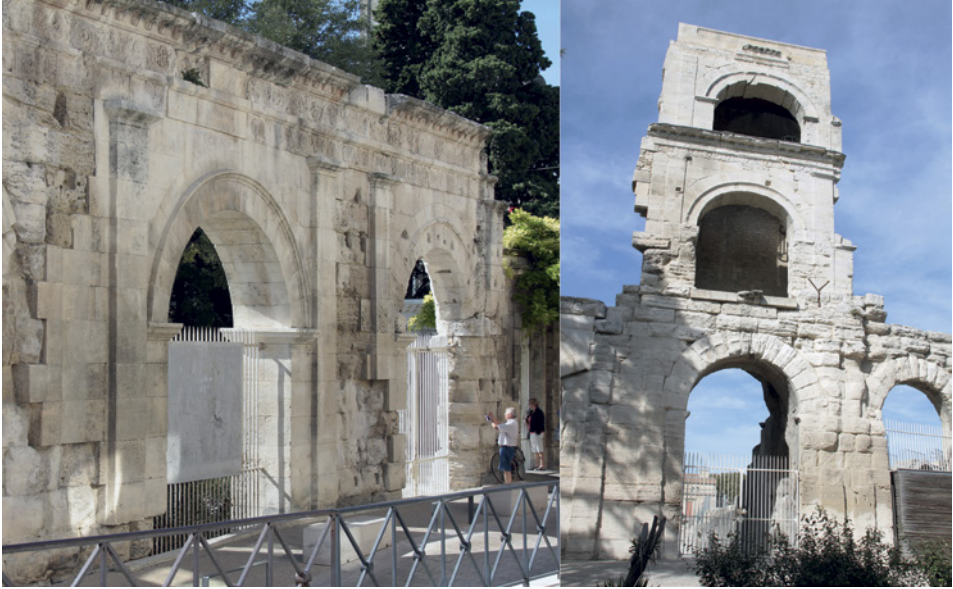
FIGURE 8.4 Left: “Arcade of Mercy”, the north side of the theatre at Arles. Right: “Tower of Roland”, the southern side of the same theatre IMAGES © F. LEMERLE
