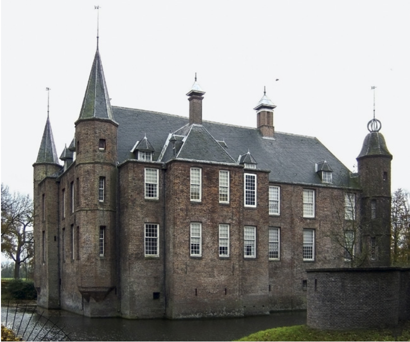
FIGURE 12.4 Zuylen Castle (Maarsse), seen from the North. Founded in the 13th century and several times enlarged and reconstructed. The northern walls date mainly from the 15th and 16th centuries
