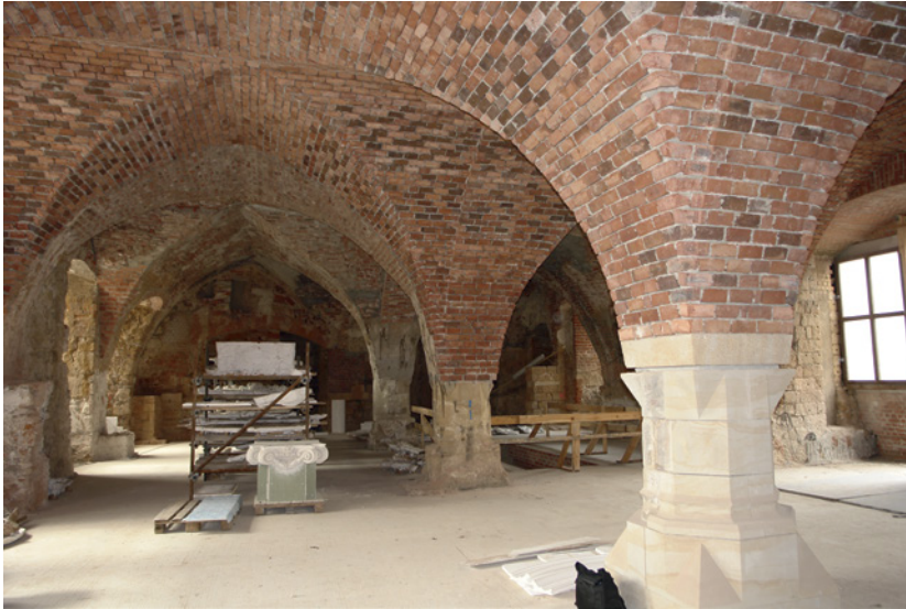
FIGURE 19.3 Arnold of Westfalen (attributed), Dresden, Schloss, ground floor hall of the east wing with its Romanesque Renaissance vault, so called “Gotische Halle” (ca. 1470–1475)
