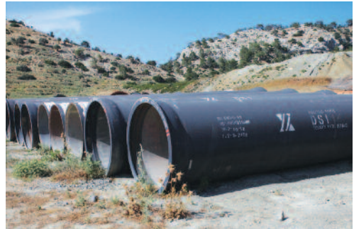
Image 6: Pipes for the distribution network in the island.
