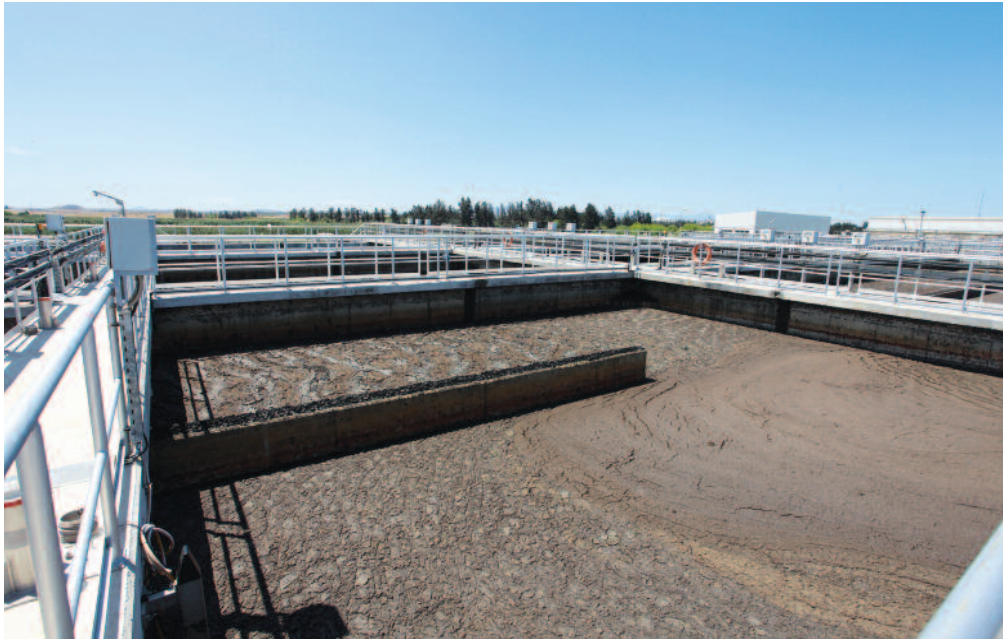
Image 1: A stabilisation pond at the New Nicosia Wastewater Treatment Plant at Mia Milia (Haspolat) outside north Nicosia.
