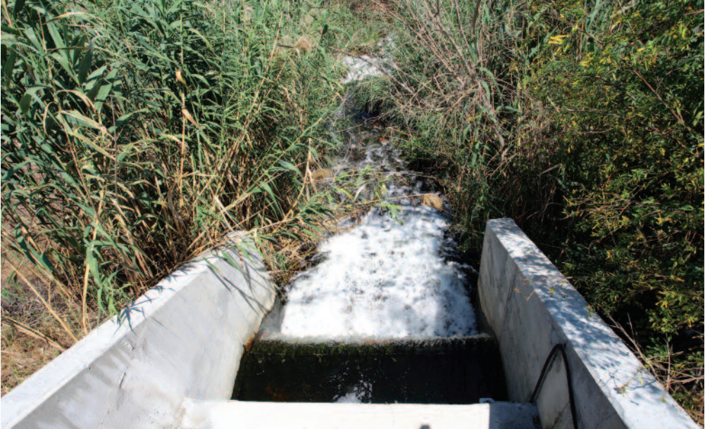
Image 2: Purified wastewater from the NNWTP spilling into ditches behind the facility.
