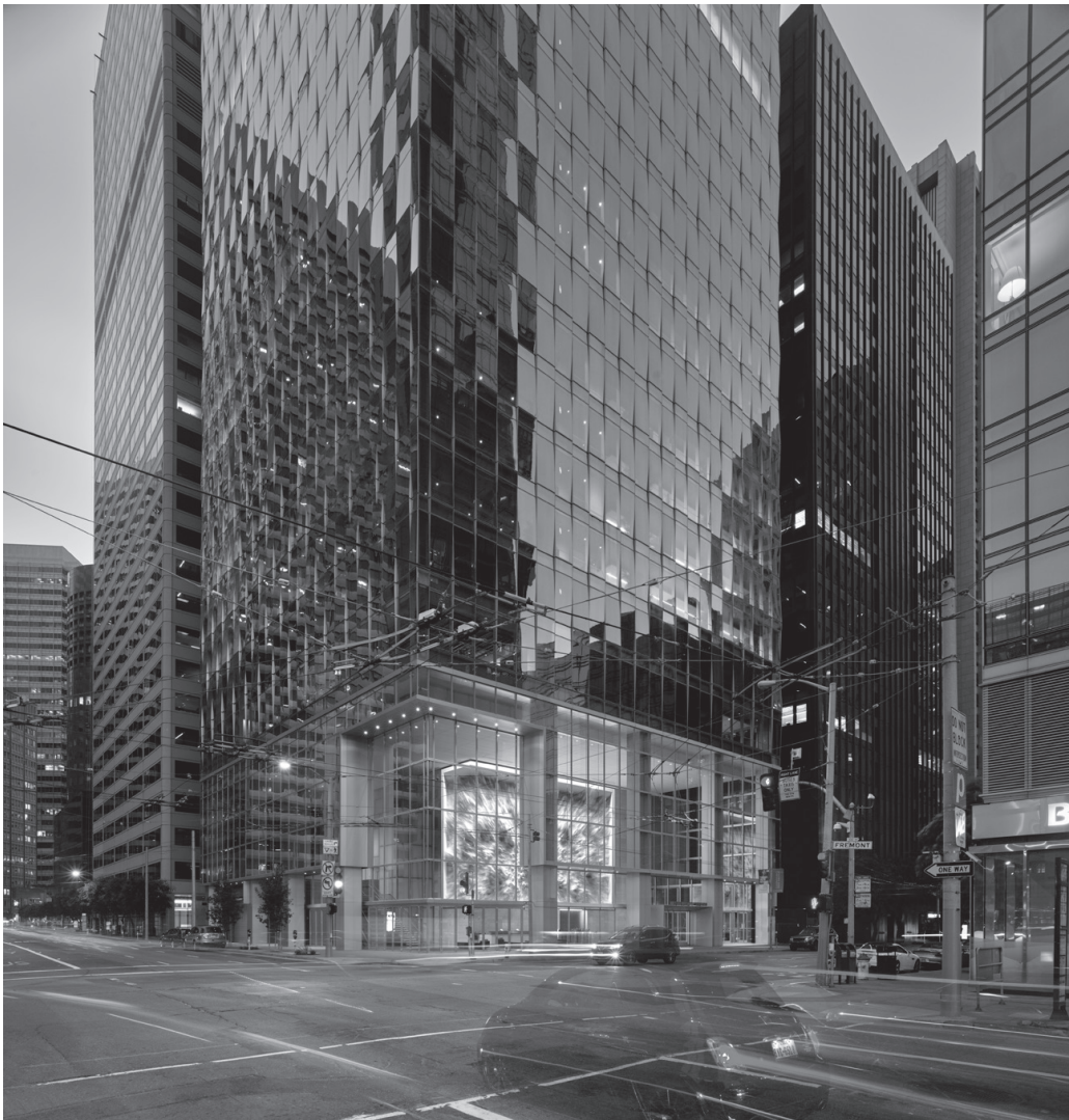
4.5: 350 Mission Street, San Francisco, a commissioned digital artwork animates a 70-by-38-foot LED screen that is visible from the street. © Skidmore, Owings & Merrill LLP | Cesar Rubio.
