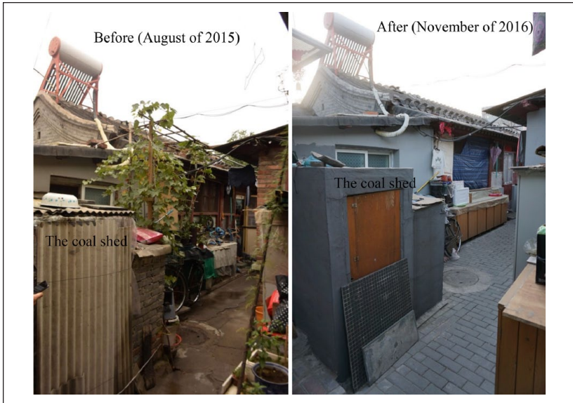
Figure 2. The Qianguaibang 4 courtyard before (provided by Ms. G) and after the renewal project.
