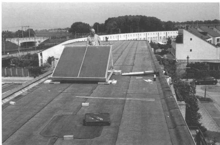
Figure 1. Installing a solar collector on a Dutch housing estate.
