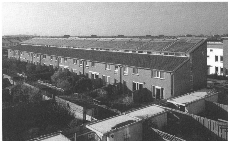
Figure 3. Solar collectors on a Dutch housing estate.
