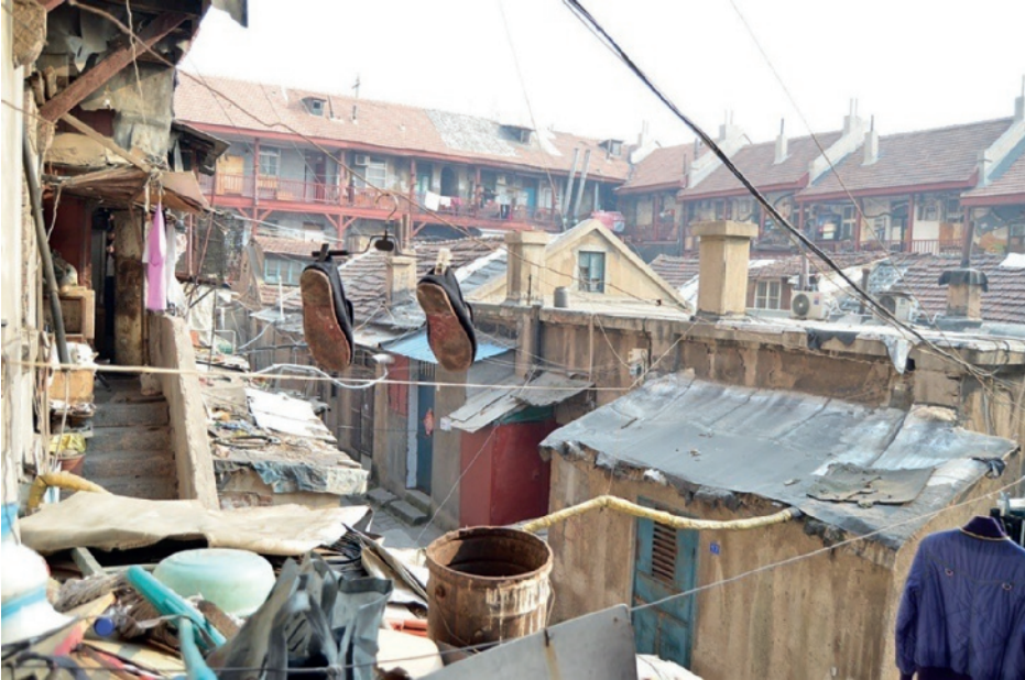
Figure 9.2 Poor living conditions in Liyuan
