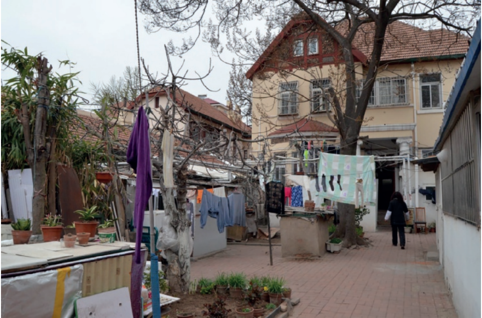
Figure 4.6 German house with illegal constructions
