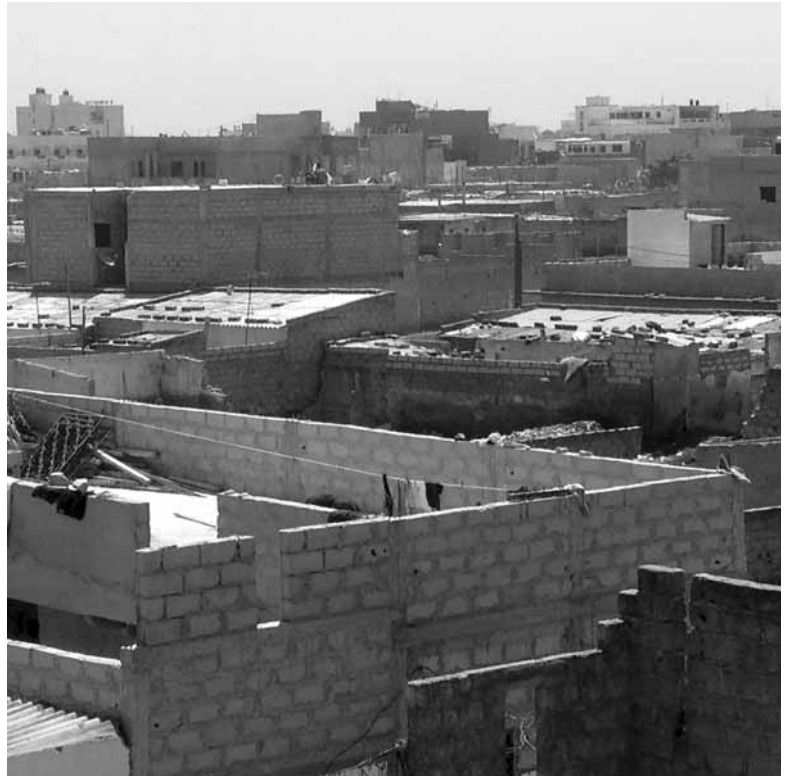
Figure 4. Unfinished houses in Keur Massar. (Photo: © Mayke Kaag)
