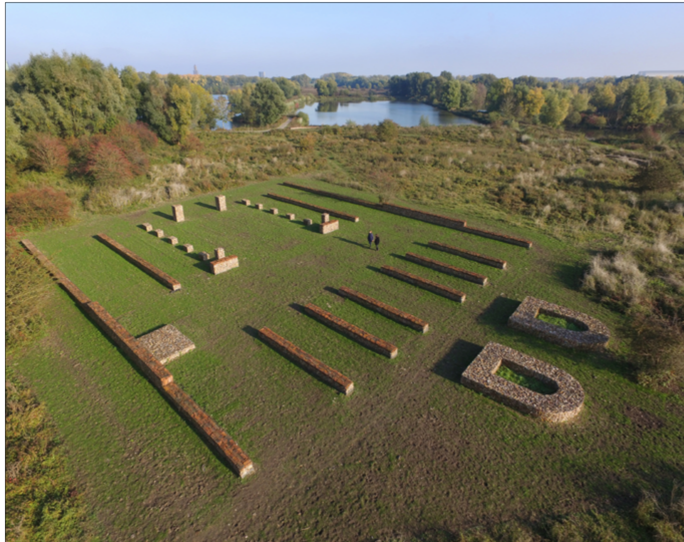
Fig. 2: At Arnhem-Meinerswijk, the walls of the headquarters and south gate have been reconstructed using gabions, with those across the river's flood-path left out. © PAUL VAN DER HEIJDEN.
