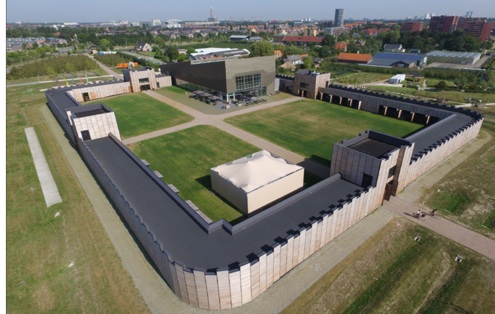
Fig. 4: Castellum Hoge Woerd at Utrecht-Leidsche Rijn: the reconstruction of the fort rampart was based on the timber-revetted ‘box type’ current in the 1st century. It was slightly widened to accommodate exhibition and education rooms, stables, offices, etc. In the foreground is the outdoor stage for the summer program. The pavilion in the background houses the ship exhibition, a theatre and a restaurant.
