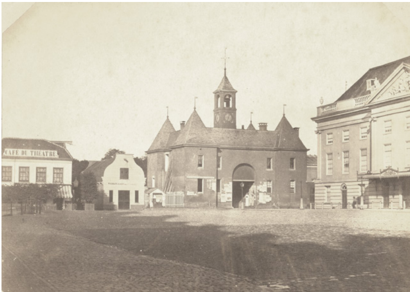
FIGURE 16.17A The former "Leidse Poort" on the Leidse Plein in Amsterdam, built 1664 by Daniel Stalpaert. Photo taken before its demolition in 1862 IMAGE © STADSARCHIEF AMSTERDAM
