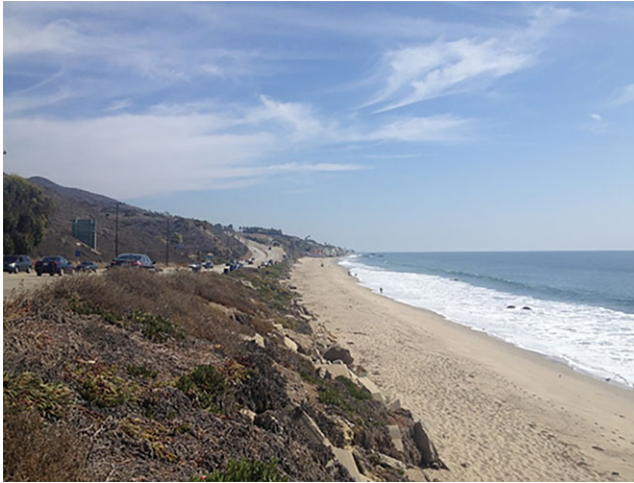
Figure 6.3. Low-lying stretch of PCH in Malibu. Beach nourishment is an important option to protect residents and infrastructure located behind beaches. However, with extreme sea level rise scenarios, some beaches cannot be augmented with nourishment, and will lose their protective capacity. In such situations, PCH could be relocated to higher ground, or elevated with fill (Photo J. Aerts).
