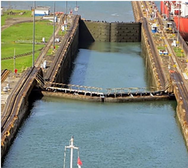
Figure L1. Sluice Lock and gates to overcome water level difference (Source: Rijkswaterstaat).
