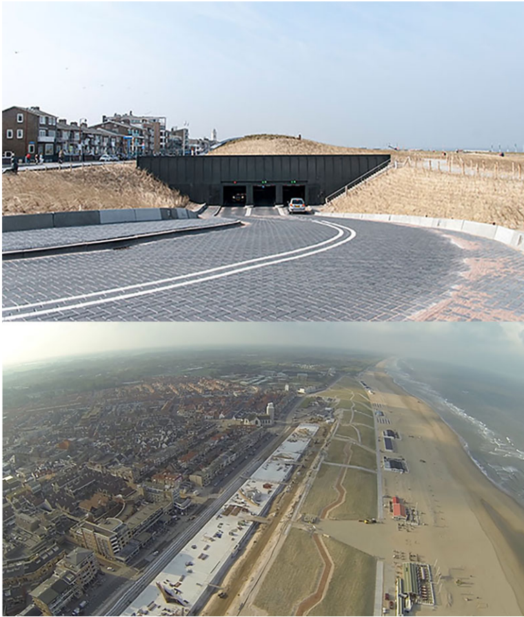
Figure 5.6. “Dike in dune” project in the City of Katwijk, the Netherlands. A reinforced concrete parking caisson was buried within a dune. The waterside of the concrete caisson of the parking facility acts as a levee, in case a storm washes away the beach and dune. As compensation for losing their view, hotel and restaurant owners can operate pavilions in the beachfront during summer months. (Source: City of Katwijk, 2018)
