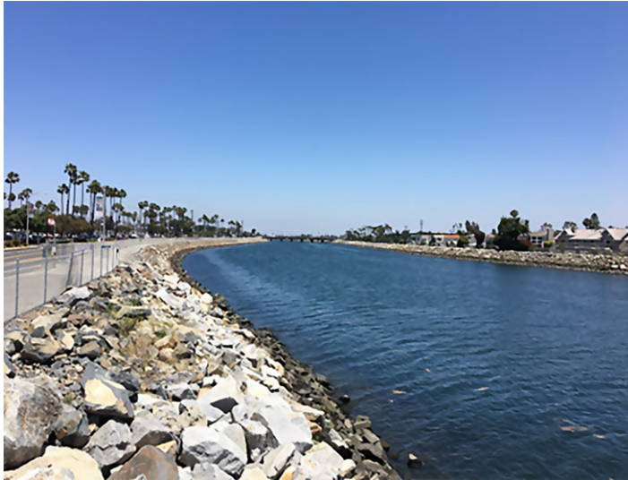
Figure 4.1. San Gabriel River near Naples, Long Beach. These levees along the river probably need an upgrade when sea levels rise in the future, and will influence (flood-) water levels in the river (Photo: J. Aerts).
