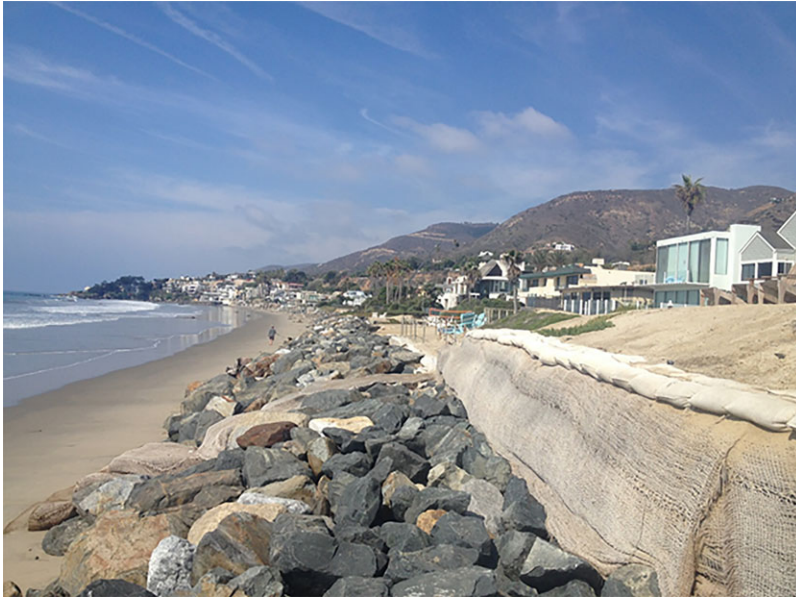
Figure 3.2. Eroded beach at Broad Beach in Malibu, protected with rip-rap. Future sea level rise may challenge the protective value of nourishment for these structures. Alternative options for adaptation include elevation of individual buildings or, eventually, managed retreat. (Photo: J. Aerts)
