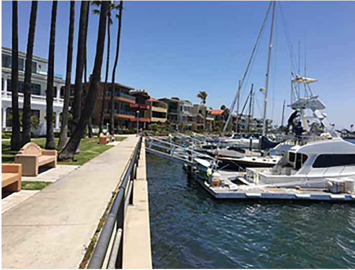
Figure 6.5. Buildings and bulkheads in Naples, Long Beach. Options for adaptation include dry and wet flood-proofing, or small flood walls where there is space. However, with accelerated sea level rise of +3–7 ft, the area will be permanently inundated, and additional flood protection is required, such as protecting the Bay area with a sluice. (Photo J. Aerts).
