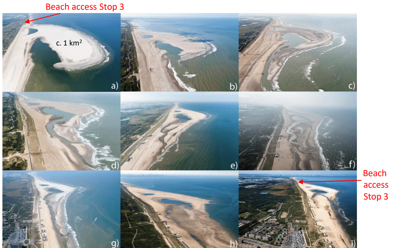
Fig. 34 – Sand Engine from the air (RWS commissioned photo series – views to the south) in 2011 (a,b), 2012 (c,d), 2013 (e), 2014 (f), 2015 (g), 2016 (h), and 2017 (i). Compilation: Rutten (2018).
