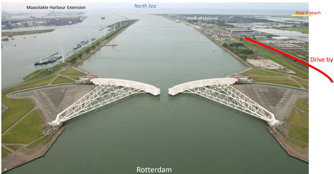
Fig. 33 'Maeslantkering' storm surge barrier closed in anticipation of storm surge 3 January 2018 (photo ANP).
