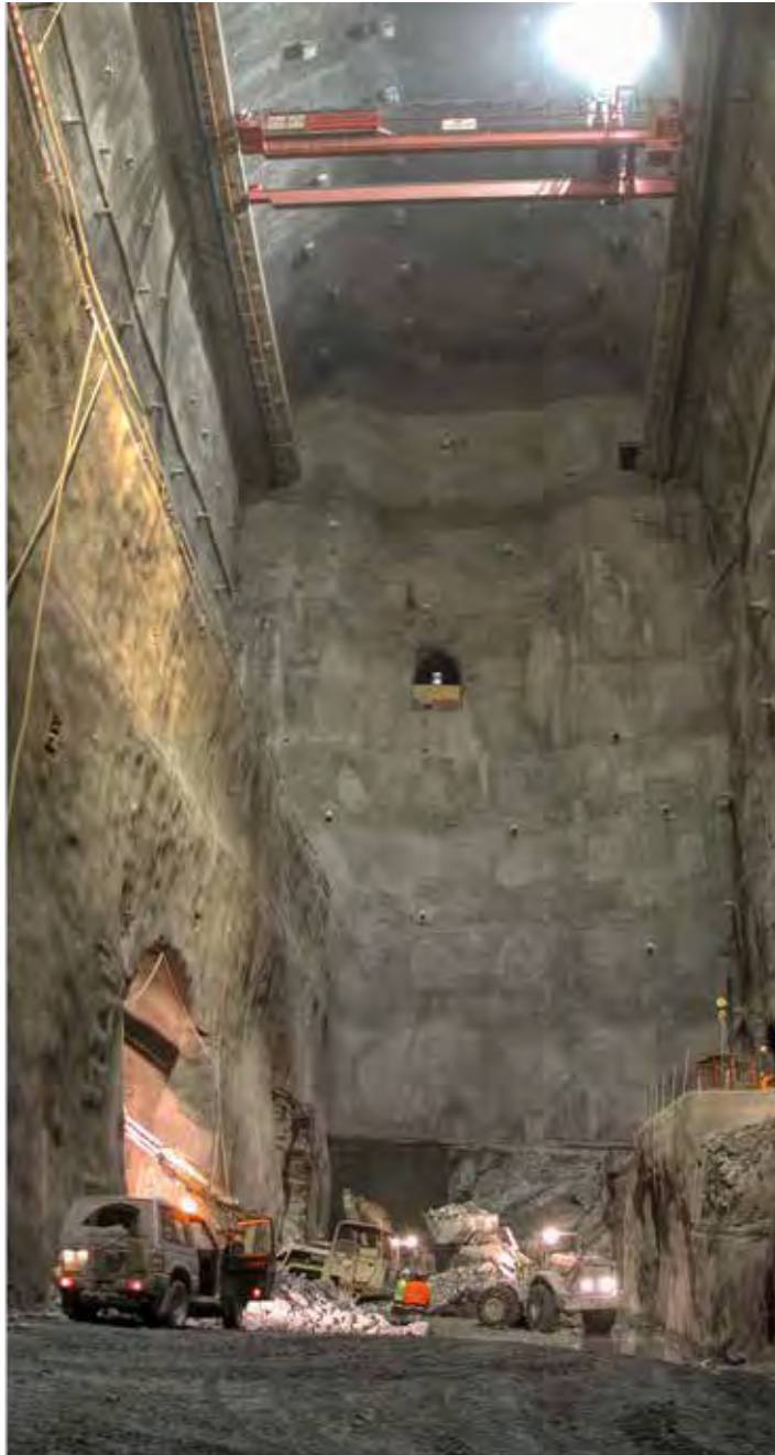
Figure 63 – Underground machine hall. Source: Illwerke VKW
