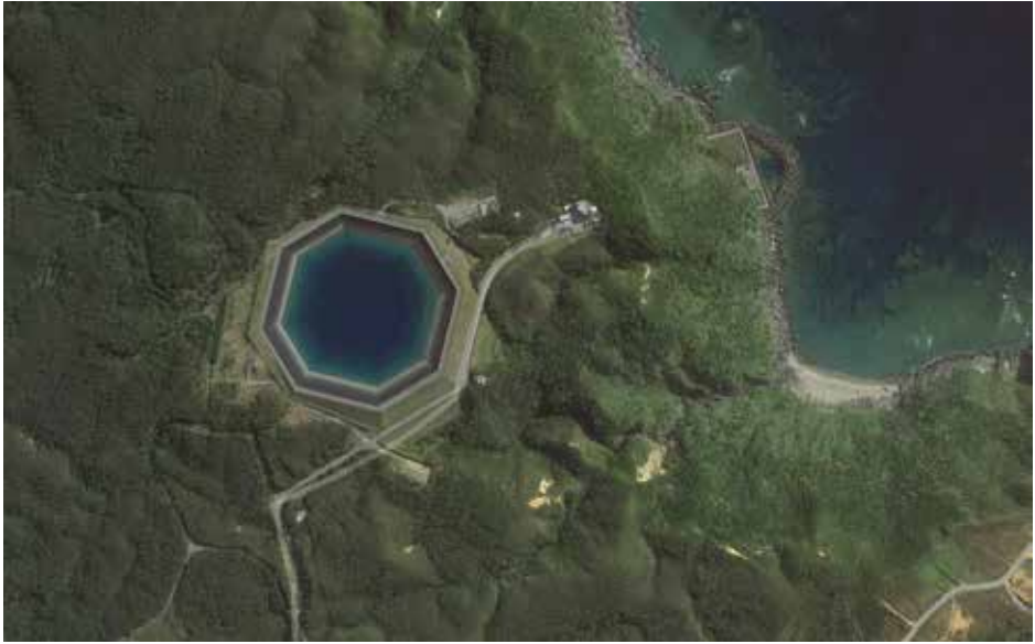
Figure 44 – Yanbaru, Okinawa, seawater PHS. The octagon-shaped upper dam is located 500 m away from the seashore at an elevation of 136 m
