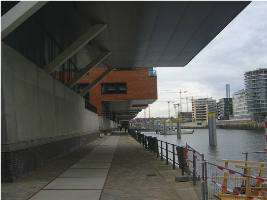
Fig. 5.1 Flood proof building in Hamburg, Germany (Source T. Raadgever)
