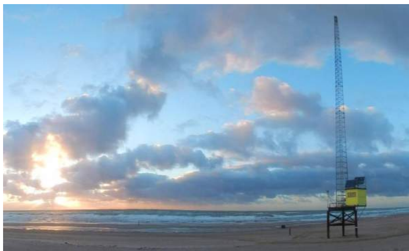
Figure 1. The Argus tower at the study site.
