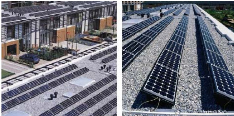
Figure 5.1 Pictures from Section K3 (Kil, 2001)
