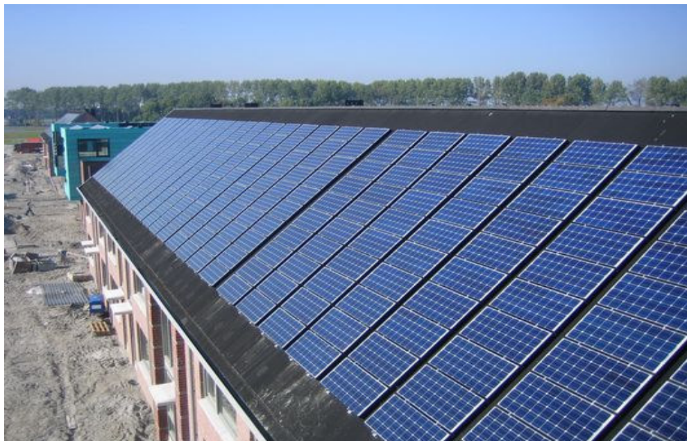
Figure 1 PV houses in Heerhugowaard
