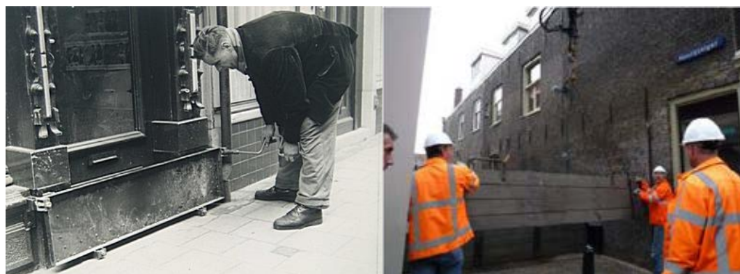
Figure 5.4: Barriers in the Voorstraat during inspections 56
