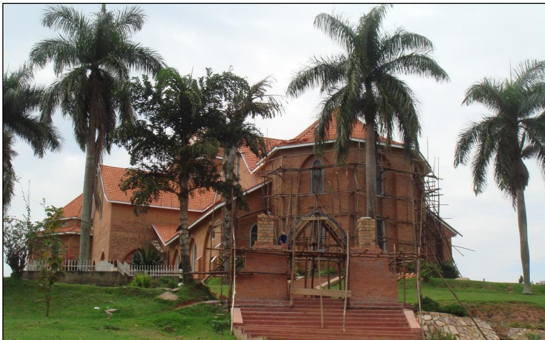
Figure A4: St. Paul's Cathedral Namirembe in Kampala, 1915-present
