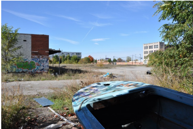
Figure 13. An abandoned boat has somehow managed to get itself into the ruins of the Packard Plant.
