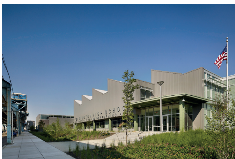
Photo 6.1 | Kensington High School manages all stormwater on site using green roofs, rain gardens and more (Focht 2013)
