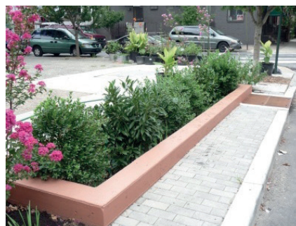
Photo 6.2 | Stormwater planters at Columbus Square Park maintained by the neighborhood community (PWD 2014)
