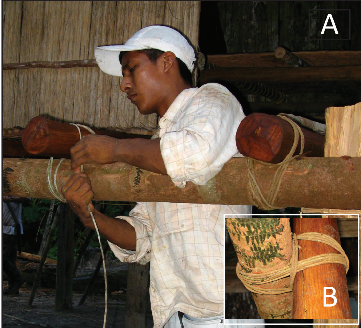
FIGURE 5. A) Field assistant Angel Hichamón (Chutty) making a knot to build a house in the Zafire Biological Station. B) Detail of the knot.
