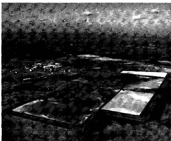
Zinc-plant in Budel, Holland; lined ponds filled with jarosite
